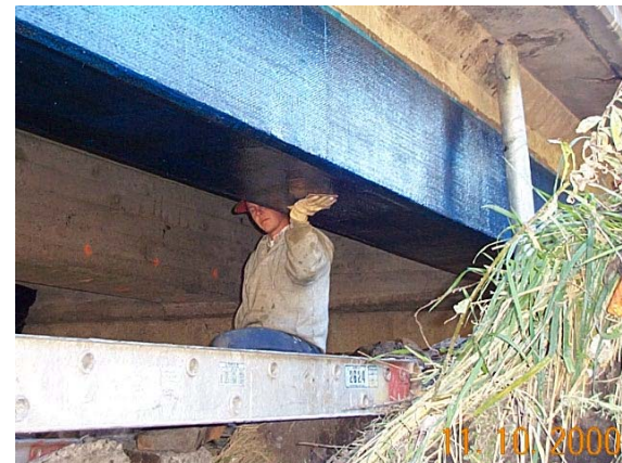
Carbon wrap concrete beam
