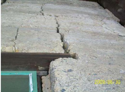
Figure 19: The crack and cavity at lintel end
