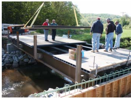
Fig 3 Goat Farm Bridge with FRP deck, Wirt County, WV
