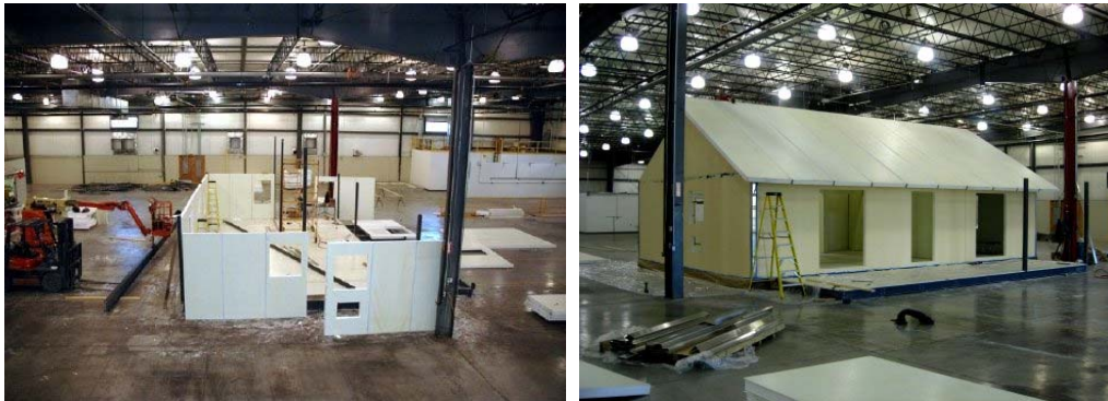
Figure 15 FRP composite house being erected at BRP Inc. manufacturing facility (2008)
