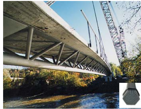
Figure 2 Kleine Emme Bridge, Switzerland, with CFRP cables in bottom chord (photo: Dr. Urs Meier)
