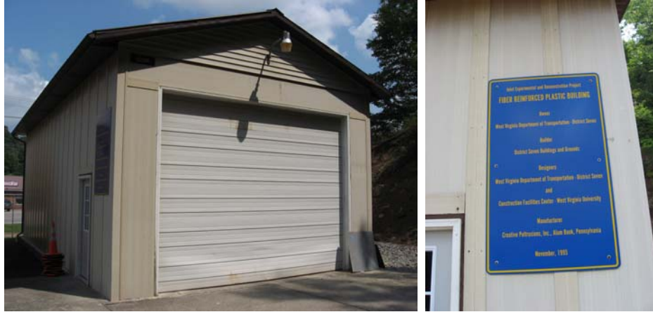
Figure 14 Multi-purpose FRP building, Weston, WV, constructed with modular FRP panels, Nov 1995 (photos taken on Aug 27, 2009)
