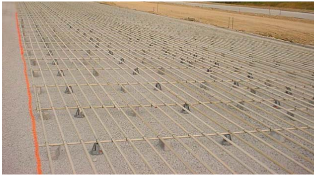
Fig 6 Pavement with FRP Rebar, WV Route 9, Martinsburg, WV
