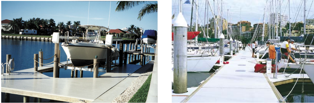
Figure 16 Marina with composite decking
