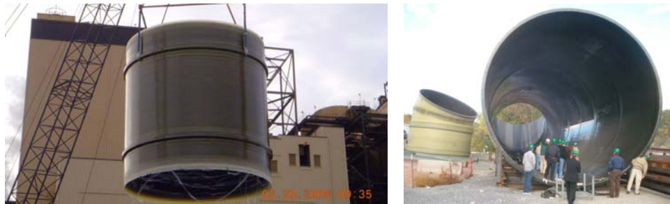
Figure 13 Large diameter FRP chimney flue liner, a) a module liner section and b) connection elbow (courtesy of International Chimney)
