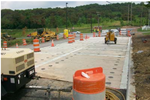
Figure 8 FRP modular panels for pavement project, before and after applying wearing surface
