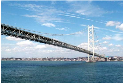
Figure 1 Akashi-Kaikyo Bridge (photo courtesy of Wikipedia.org)
