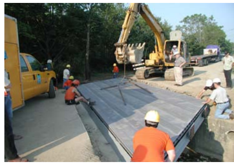
Fig 4 Pleasant Plain Road Bridge, Montgomery County, Ohio
