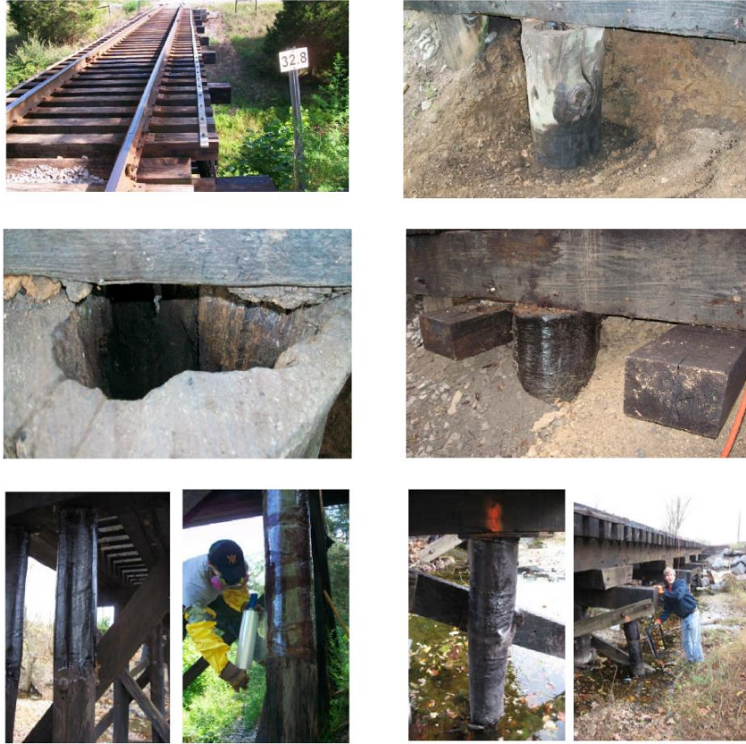
Figure 18 Retrofitting of railroad bridges using FRP wraps, SBVR, Moorefield, WV (July 2010)
