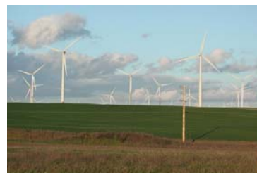
Wind Turbines – 21,000 MW capacity in the U.S.
