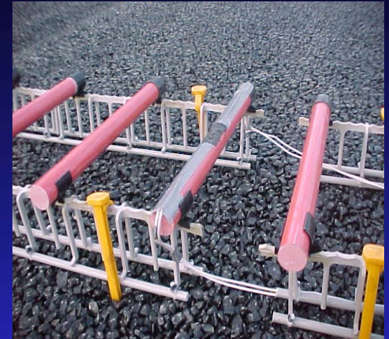
Close-up of instrumented FRP dowel bars
