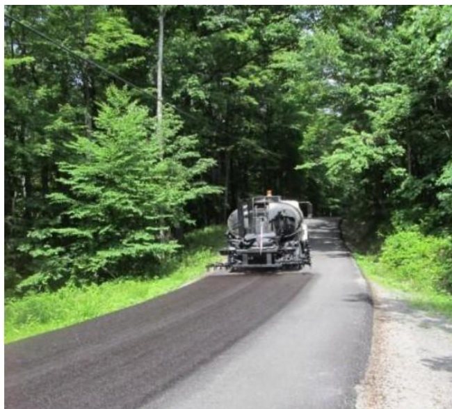
Figure 30. Fog Seal Application at Quarry Run Road Project
