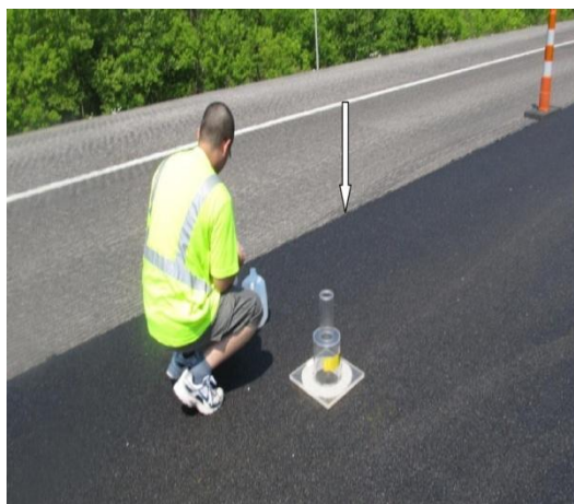
Figure 28. Field Permeability Test Conducted at I-79 Project
