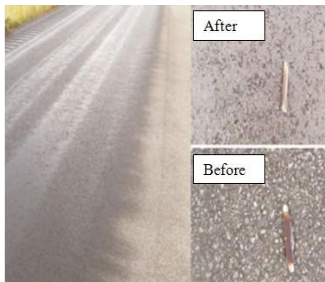
Figure 31. Mon-Fayette Pavement Surface before and after the Fog Seal
